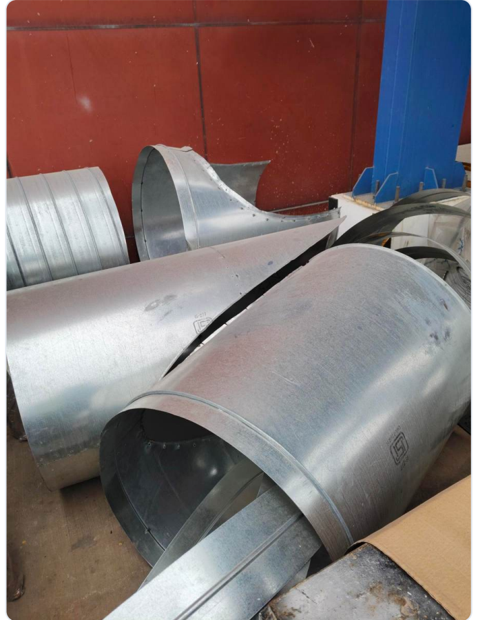
Photo 2: Site photograph, staged sections in marked lanes | Captured on site, geotagged
